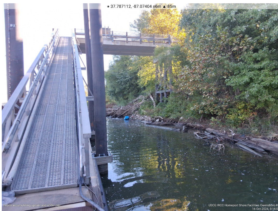
Photo 6 Debris accumulating upriver and under pier. View of gangway connecting pier and floating dock.
